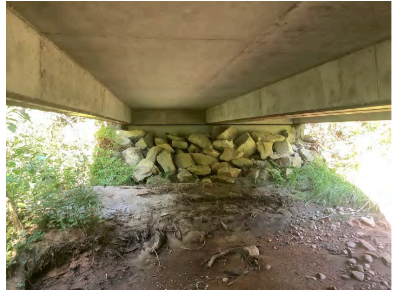
Right Bank Abutment when facing downstream
