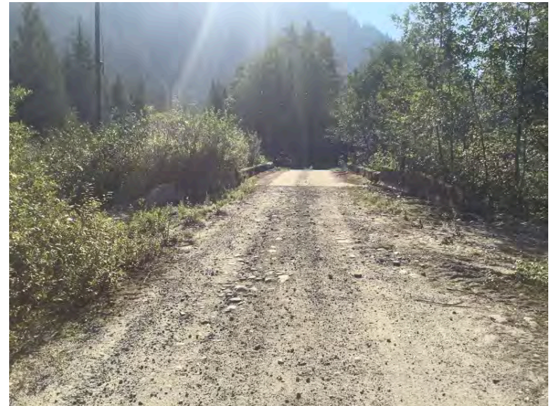
Approach from Right Bank when facing downstream
