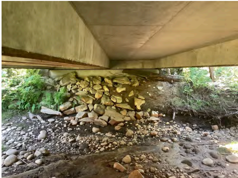
Left Bank Abutment when facing downstream
